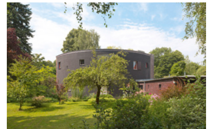
> Residential building by Bruno Taut in Dahlewitz
